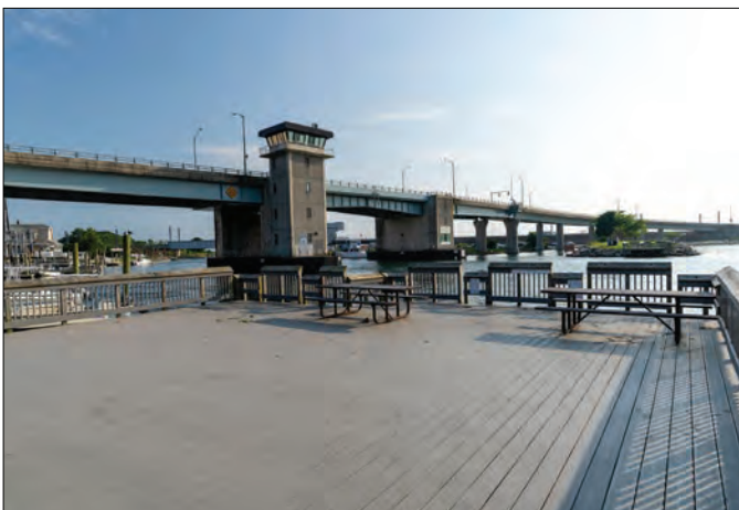
Head Over The Bridge To Niantic!
